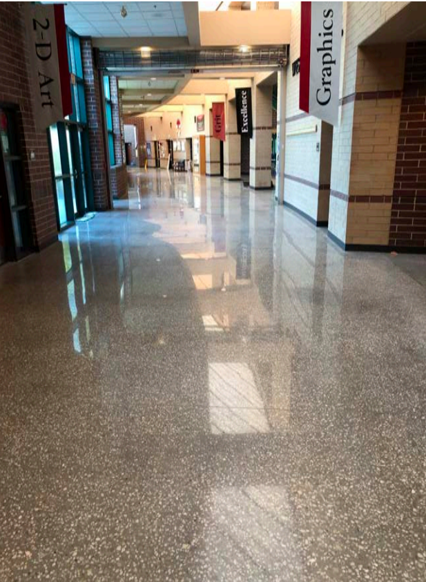
Scope: Remove VCT tile and replace with polished concrete, repair pool deck, construct elevator at LES
